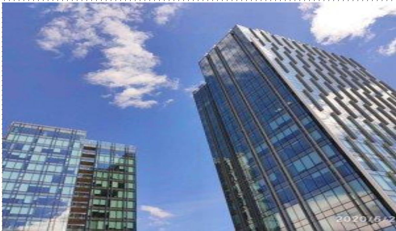
BC AURA, 2nd LINE OF CONSTRUCTION- NUR SULTAN
